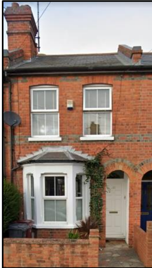
31 Chester Street, Caversham (c.2022)
